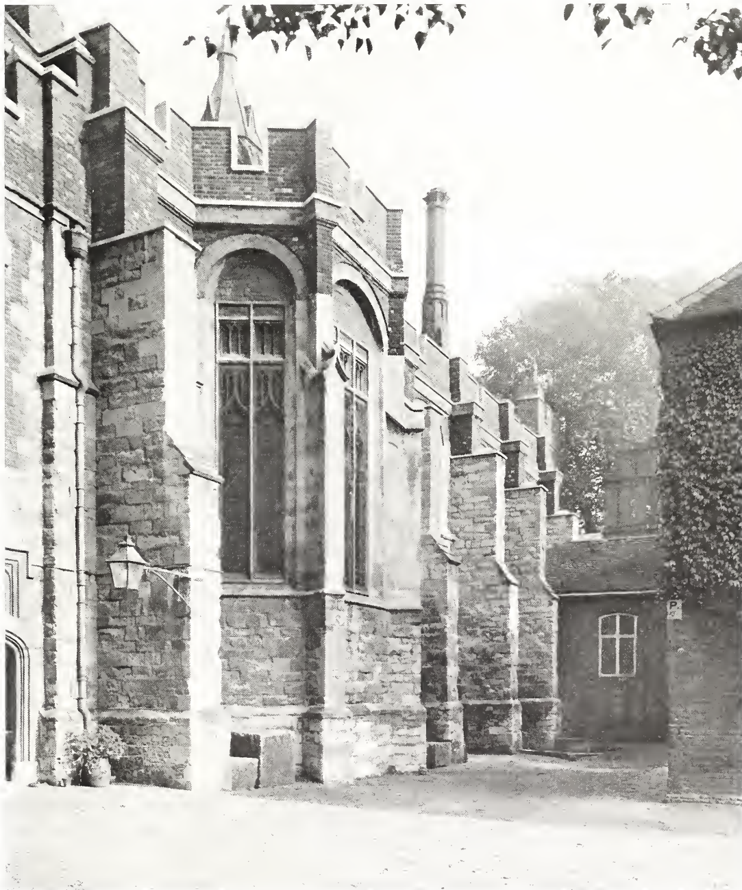
SOUTH FACE OF THE HALL.
